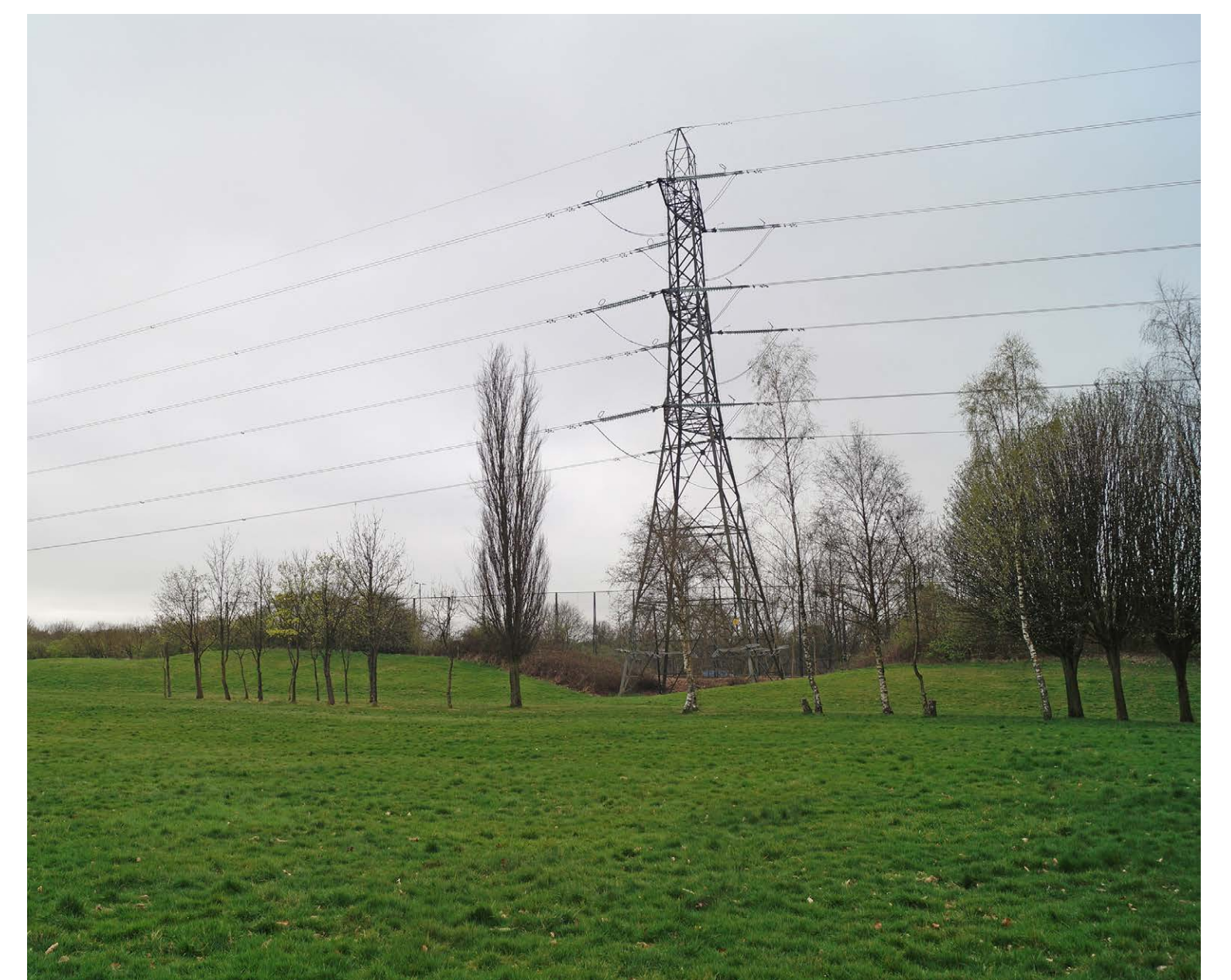
Western Boundary: Existing utilities will influence future development and we need to take account of noise and air quality issues near the M5.
